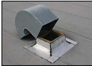
This goose-neck was secured with two screws. Failure lead to significant water entry into the building Source - FEMA
