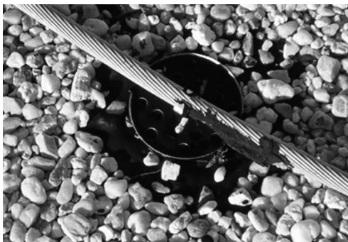
Conductor secured with clip adhered to cover
