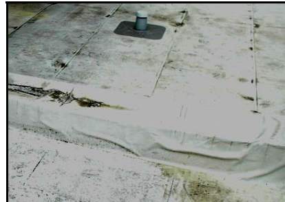
Ductwork installed under roof cover
