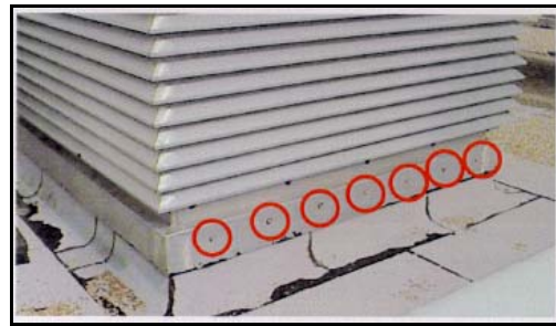
Adequate securement Source - FEMA
