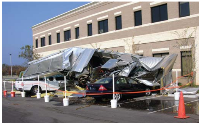
18,000 lb HVAC unit secured to curb with 16 straps, one screw per strap. Wind speed 85-90 mph Source - FEMA
