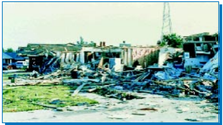
Hurricane Andrew tornado damage, LaPlace, LA/NOAA
